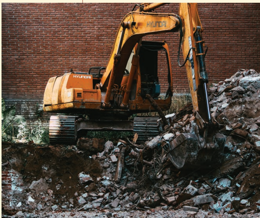
A history of construction activity at an urban site oftentimes results in compacted soil that contains both debris and contaminants. Photo by Francisco Andreotti
