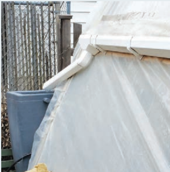
A high tunnel with attached rain gutters and a 50-gallon rain barrel. Photo by Cherry Flowers, Holistic Health Farms
